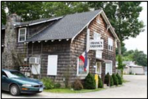
Store with apartment above
