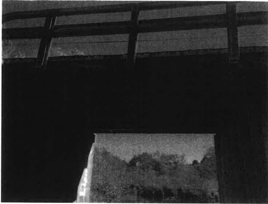
Photo 9 – Downstream Face (Looking Upstream)
